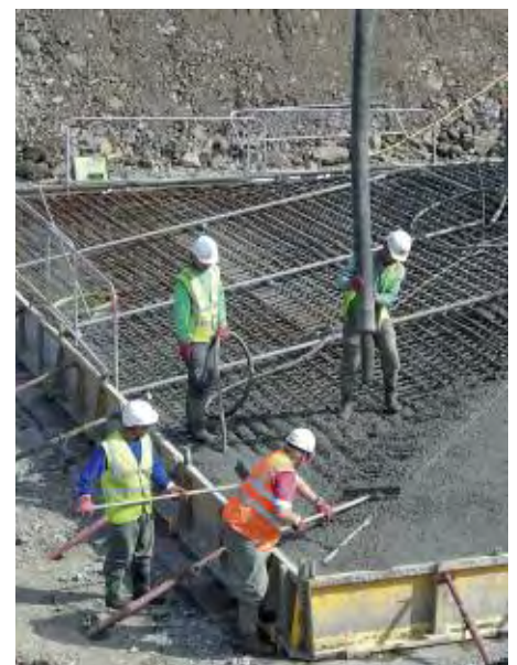
Phoenix Portland-fly ash cement being used at Whitelee windfarm, Scotland
